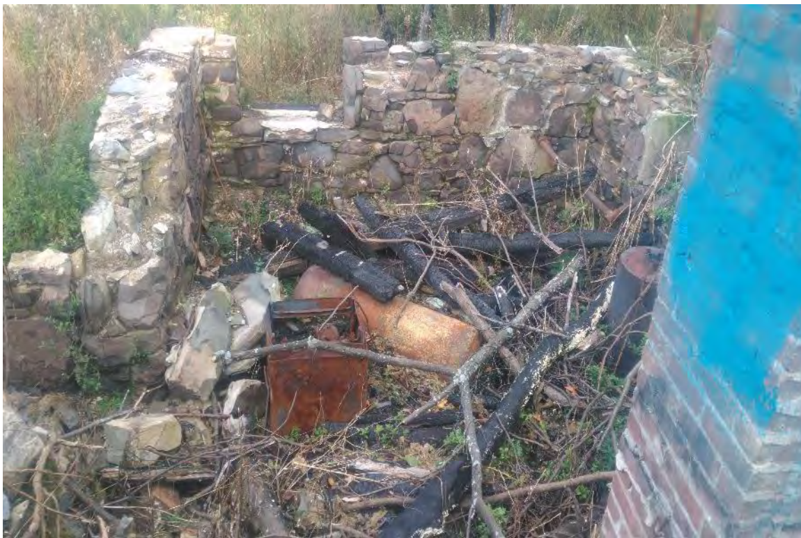
Photo 51: The wooden superstructure of the N. W. Howell house is no longer extant, and only the mortared stone foundation and brick chimney remain. View to the east.
