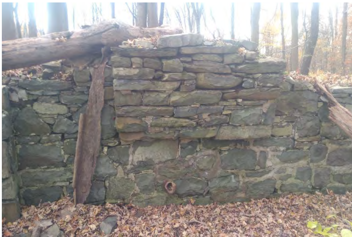
Photo 23: Ceramic pipes are located within the mortared stone wall of the farmhouse foundation. View to the south.
